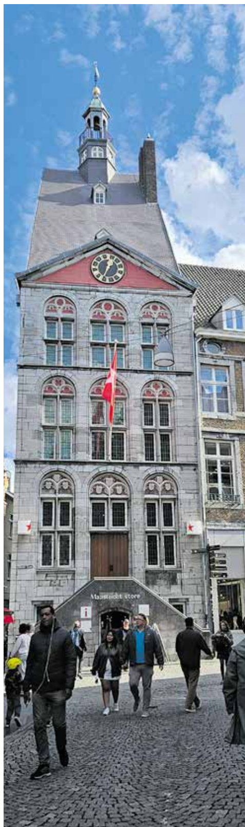
The ‘Dinghuis’, the former court building
